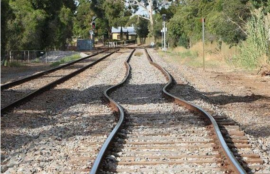
Figure 0-2 Thermal Expansion in Railway Track [8]
