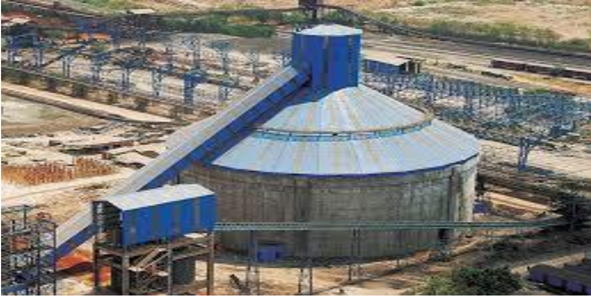
Figure 0-1 View of Cement industry showing Pan Conveyor and Clinker Yard [1]
